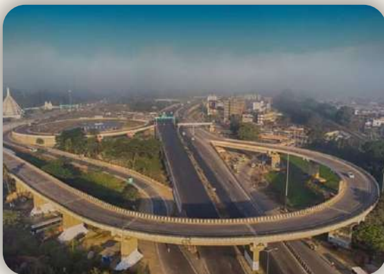
JALUKBARI FLYOVER "7KM"
