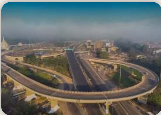
JALUKBARI FLYOVER “7KM”
